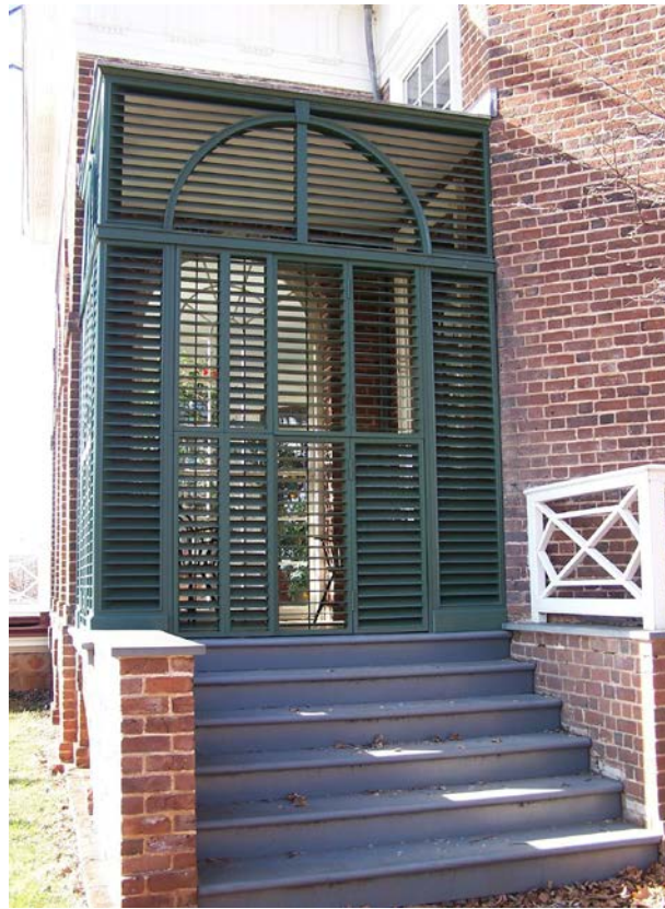
Fig. 1.28 Porticoes outside Jefferson's bedroom at Monticello, installed in 1809.
